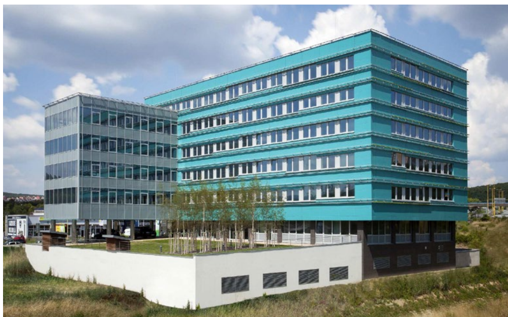
EcoPoint Office Center Košice SEMOS, spol. s r.o. Prešov
